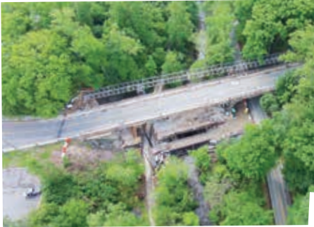
Carroll Avenue Bridge rehab.
