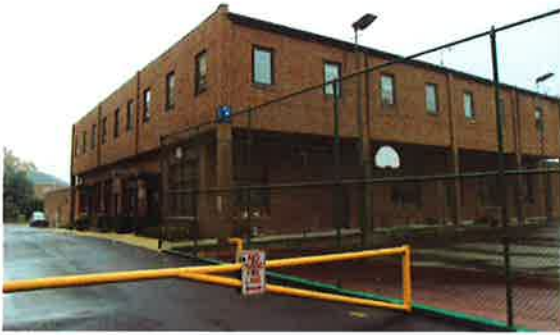
Figure 1: Existing Health Science Building
