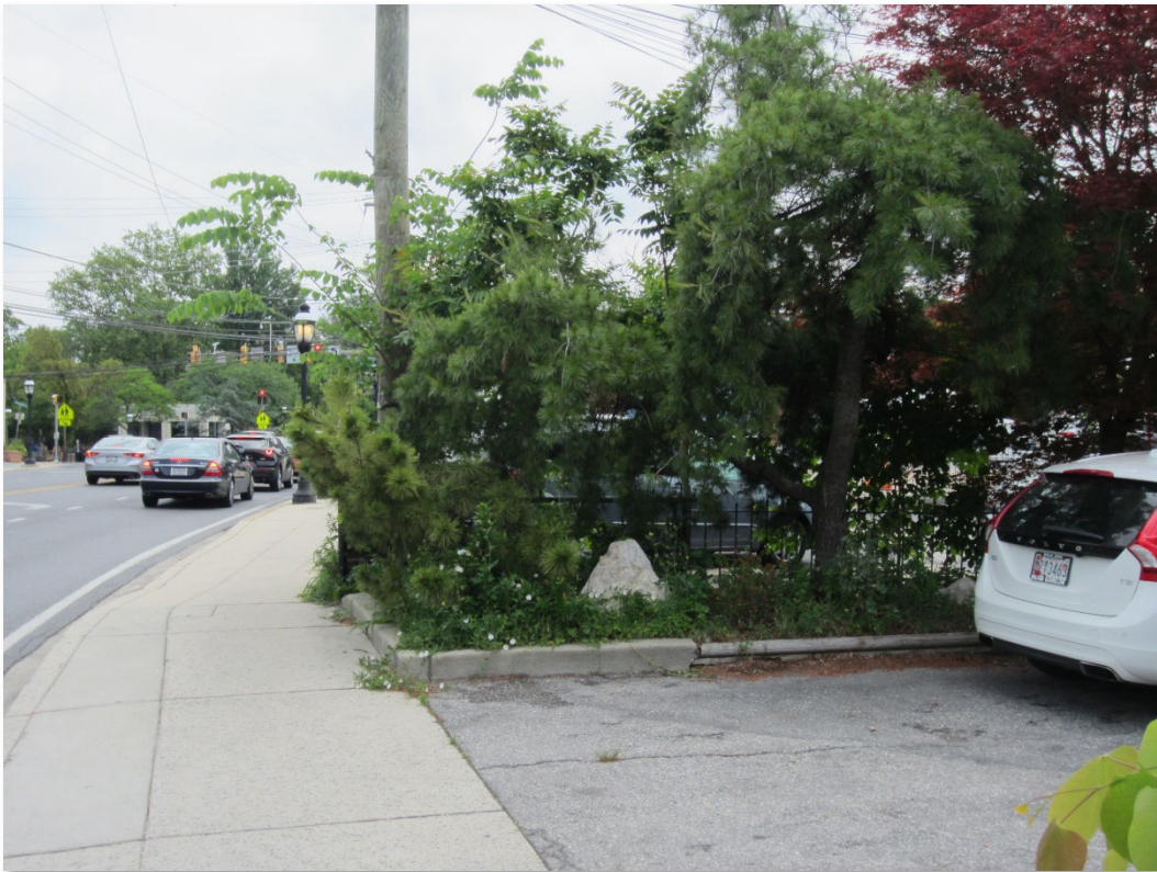
Picture 2 – Intersection Sight Triangle Opposite View Blocked by Vegetation on Adjacent Lot
