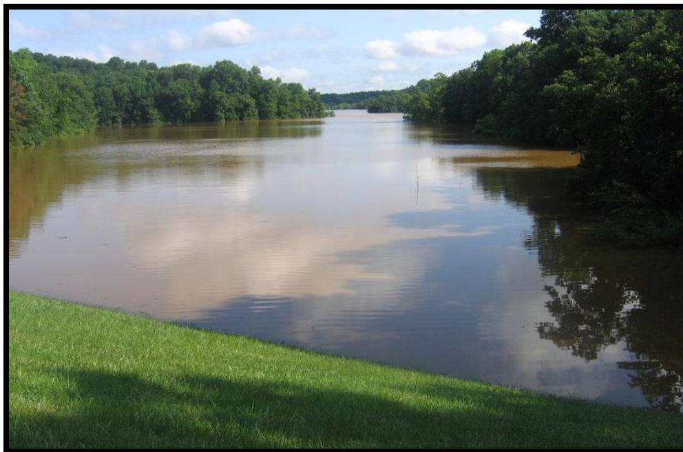
Figure 78: Lake Needwood Dam
