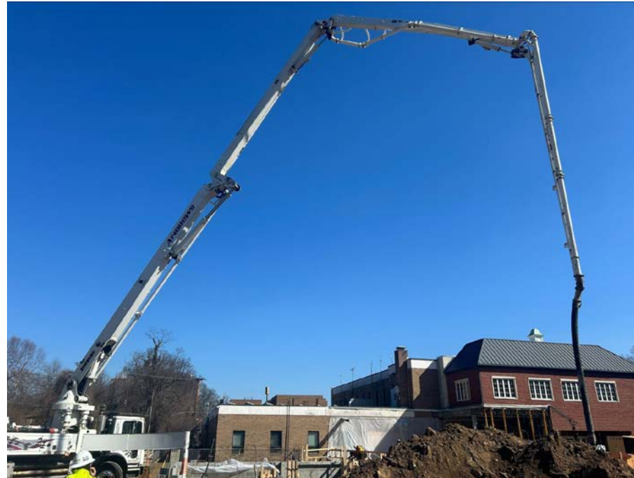
A concrete boom truck pouring the void space inside newly stacked cinder block walls solid (above). Stacked cinder block walls and rebar wait for additional formwork and concrete (right).
