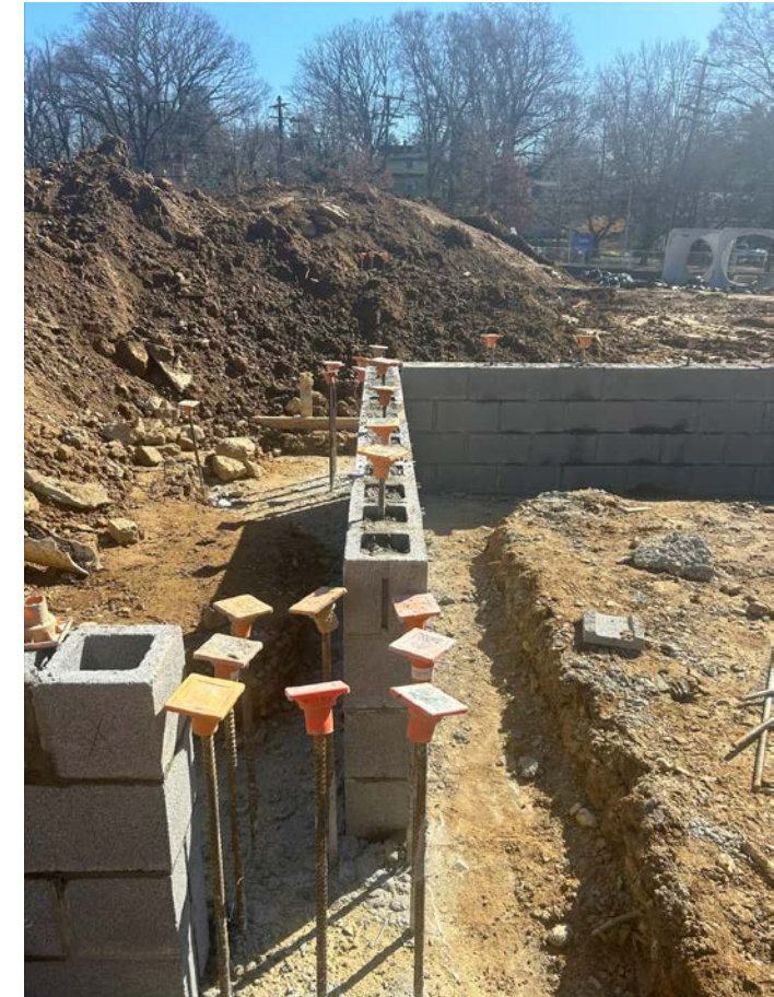
A concrete boom truck pouring the void space inside newly stacked cinder block walls solid (above). Stacked cinder block walls and rebar wait for additional formwork and concrete (right).
