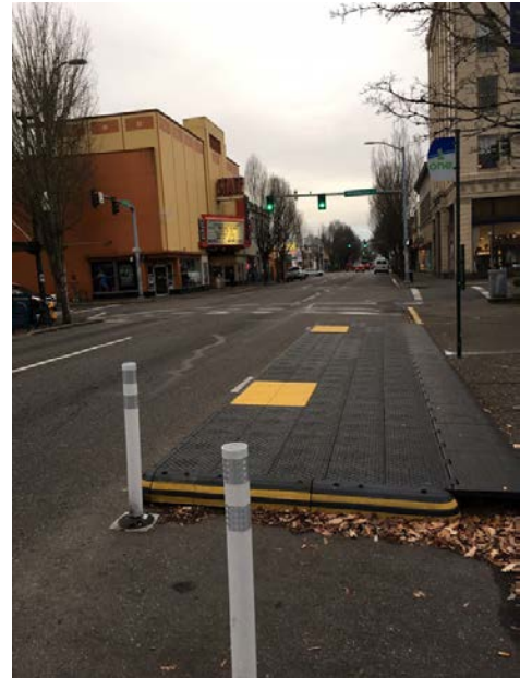
Figure 3-8: Snap In Place Plastic Bus Bulb in Olympia, WA
