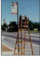
PLACE LADDER NEXT TO POLE ON A SECURE LEVEL SURFACE.
