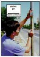
MEASURE AND MARK POLE FOR CONNECT MOUNTAINS HEIGHT TURE SHOULD BE LOW ENOUGH FOR WHEELCHAM ACCESS.
