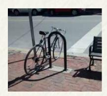
NARROW BASE HOOP RACK INSTALLED TOO CLOSE TO BENCH AND U-CHANNEL IN BRICK ON CARROLL AVENUE (SURFACE MOUNT ON CONCRETE BASE).
