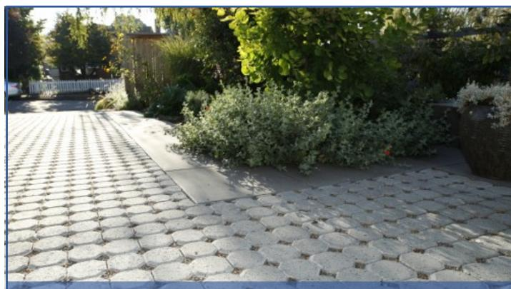
Permeable paving systems allow infiltration of water.
