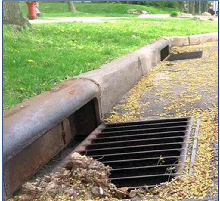
The public storm drain system is designed to carry stormwater away from developed areas and prevent flooding.
