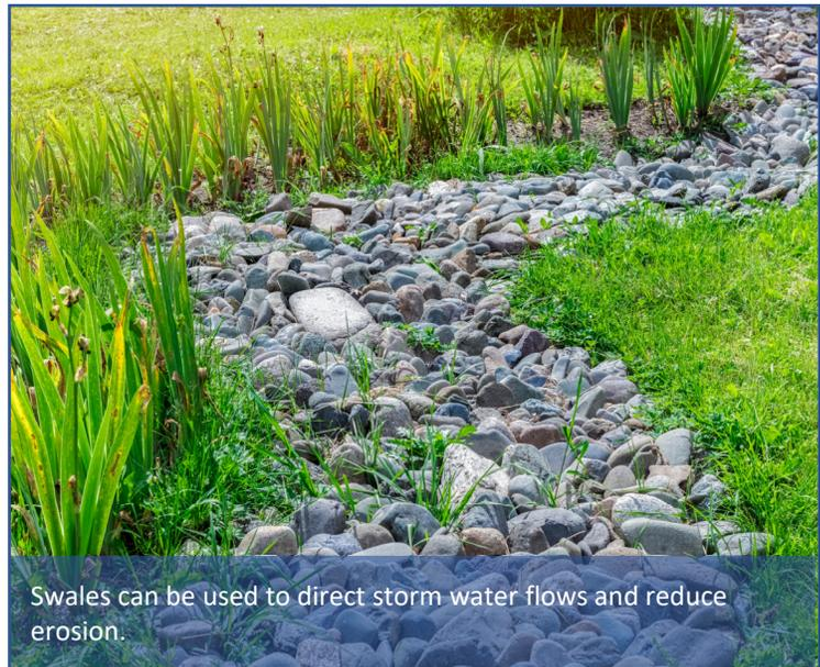
Swales can be used to direct storm water flows and reduce erosion.
