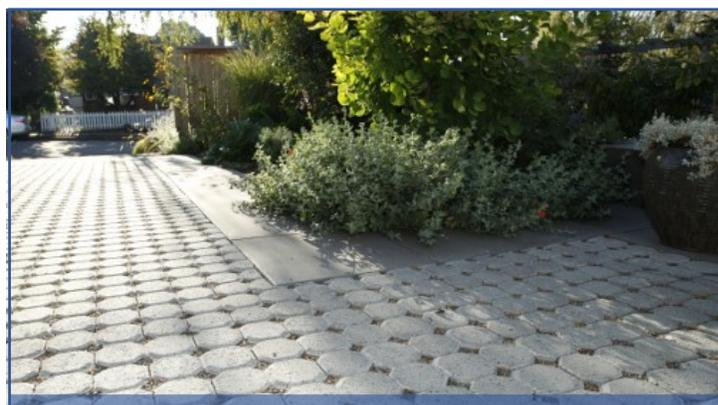
Permeable paving systems allow infiltration of water.
