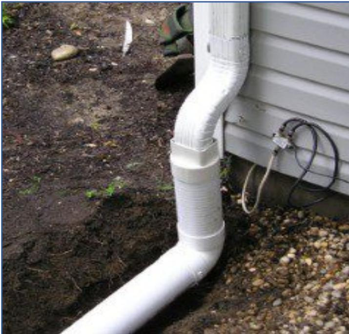
Leader pipes can be used to extend downspouts beyond building foundations.
