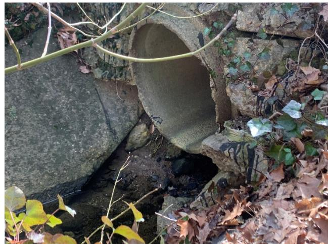
Photo 31 – Structure #881 is cracked on bottom causing erosion under pipe
