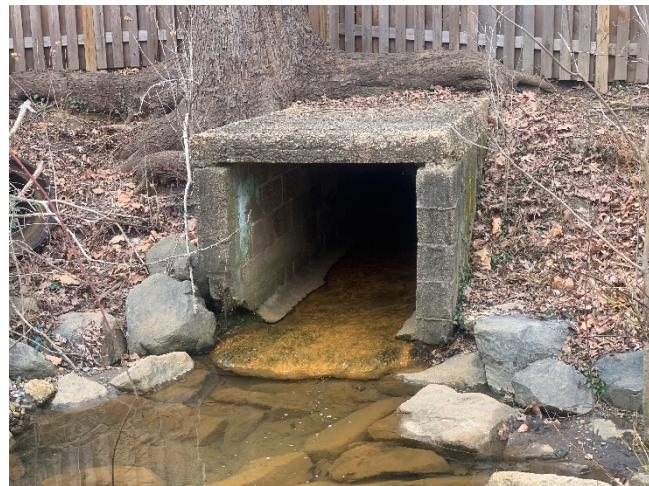
Photo 27 – Structure #212 – Corner of outfall broken
