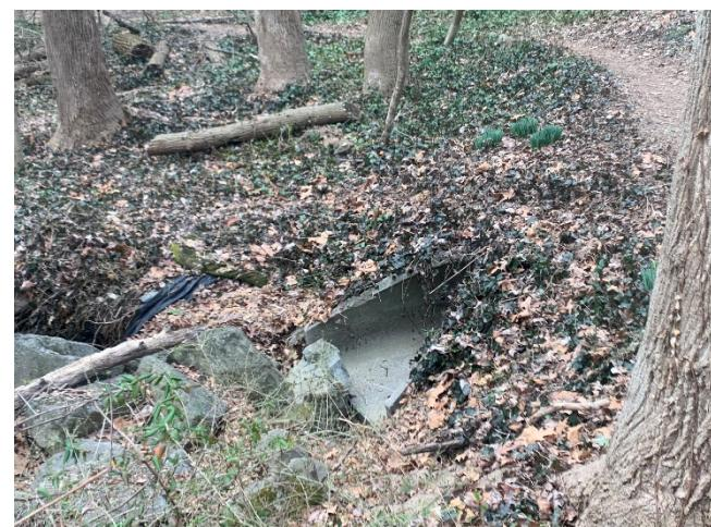
Photo 43 – Structure #1080: Riprap partially obstructing flow
