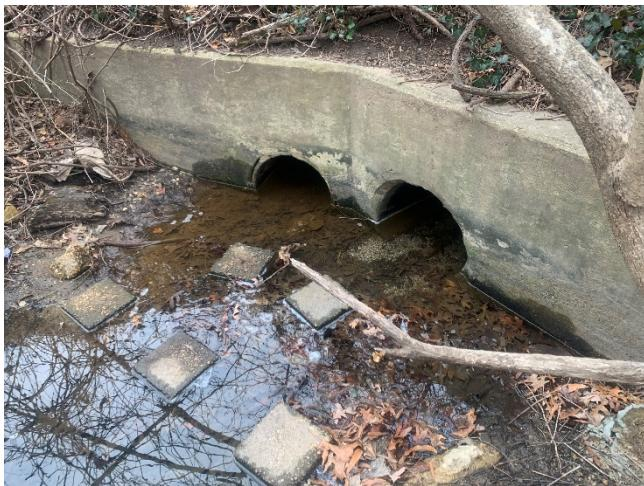
Photo 26 – Structure #71: Outfall 60% clogged with sediment
