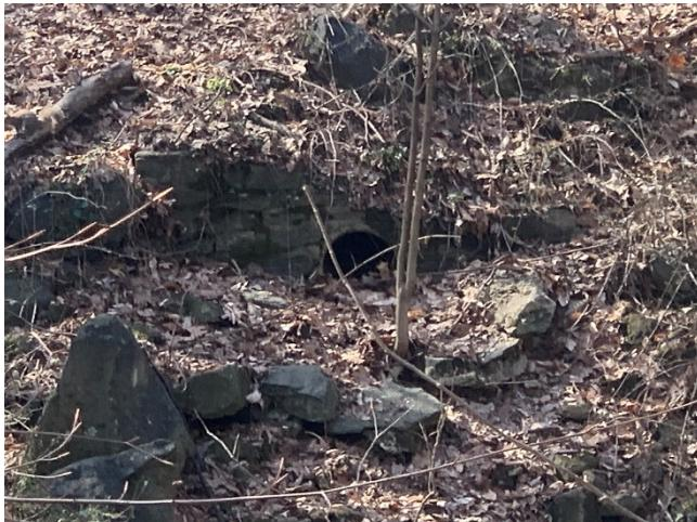
Photo 40 – Structure #1004: Outfall filled 35 percent with sediment and debris
