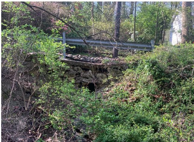
Photo 34 – Structure #962: Road edge and concrete section of the outfall pipe is failing and bank erosion downstream
