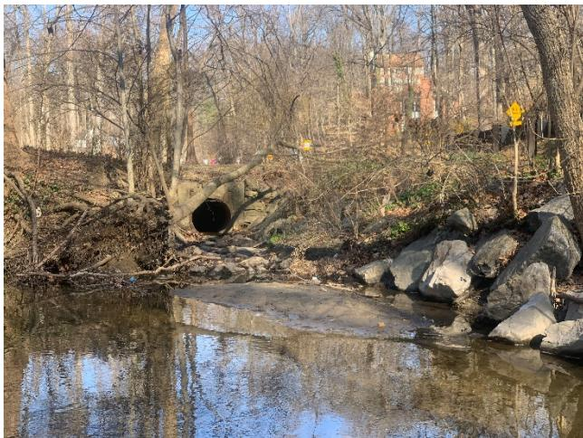
Photo 32 – Structure #930: Outfall cracked on bottom causing erosion under pipe
