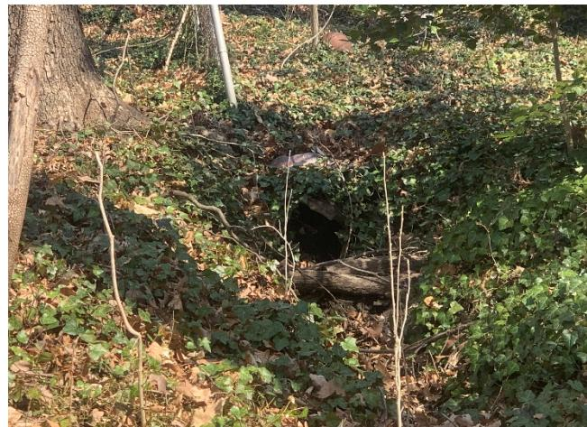
Photo 35 – Structure # 973: Outfall overgrown with vegetation and pipe broken
