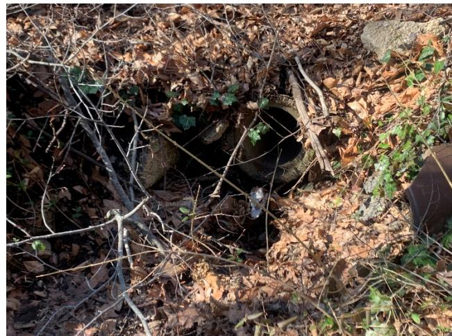
Photo 33 – Structure #960: Outfall has erosion under the pipe, has headcut and eroded banks leading to stream
