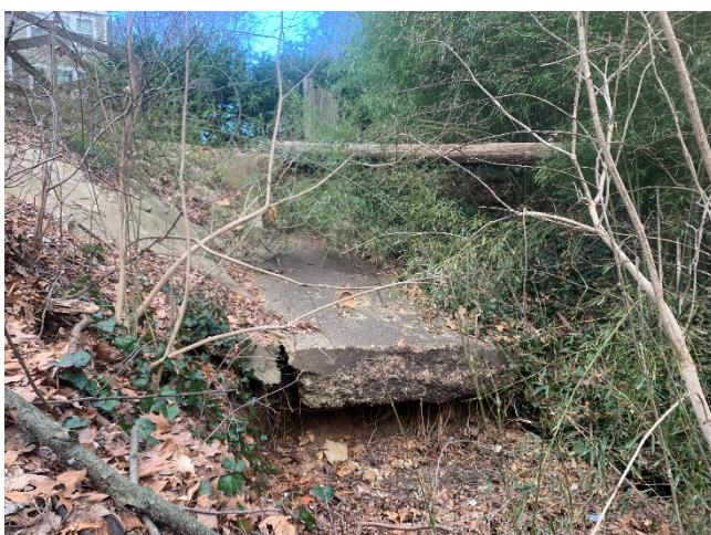
Photo 42 – Structure #1028: End of concrete channel undermined, 2-foot drop to channel along with eroded banks
