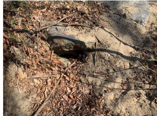
Photo 41 – Structure #1005: Outfall 95% full of sediment
