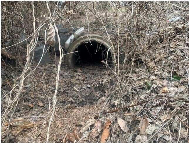
Photo 28 – Structure #273 – Outfall filled with sediment
