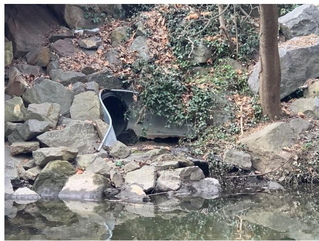
Photo 37 – Structure #983: Base is eroded and wingwall is cracked
