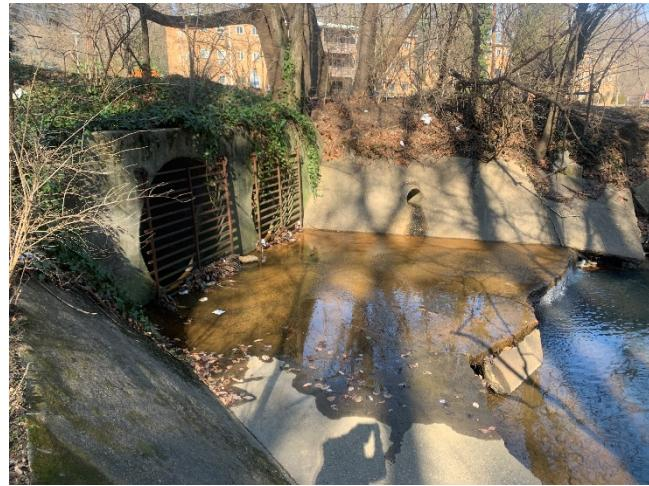
Photo 29 – Structure #289 & #290: Concrete apron cracked and undermined with deep scour pool; wingwall is cracked
