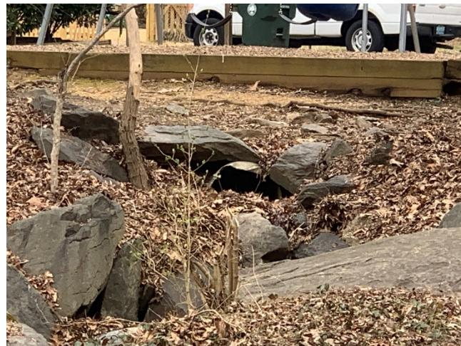
Photo 45 – Structure #1153: Outfall pipe is crushed and 40% filled with sediment
