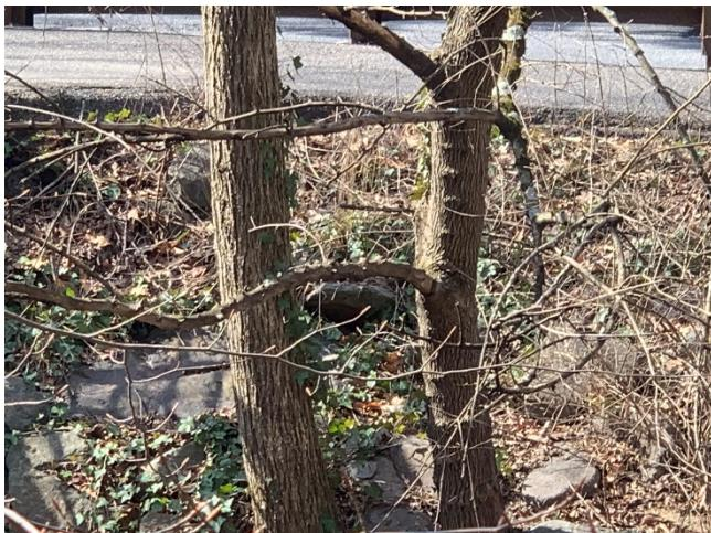
Photo 30 - Structure #854: Outfall is filled with sediment and leaf matter
