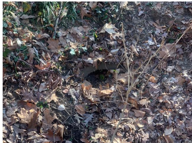
Photo 39 – Structure # 991: Outfall filled 95 percent with sediment and debris
