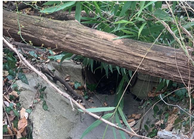
Photo 25 – Structure #60: Concrete outfall cracked and failing
