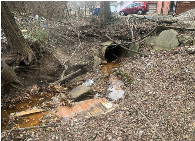
Photo 24 – Structure #55: Failing concrete apron with minor undermining and high bank erosion downstream
