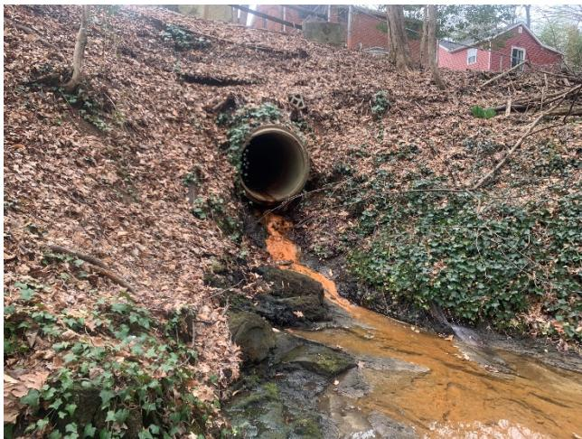
Photo 44 – Structure #1107: Crack in the pipe causing water to flow under the outfall causing erosion beneath the pipe
