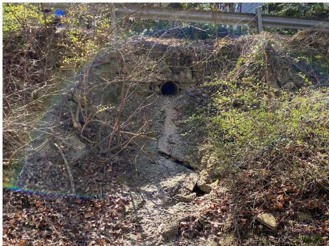
Photo 22 – Structure #962: Road edge and concrete section of the outfall pipe is failing and bank erosion downstream
