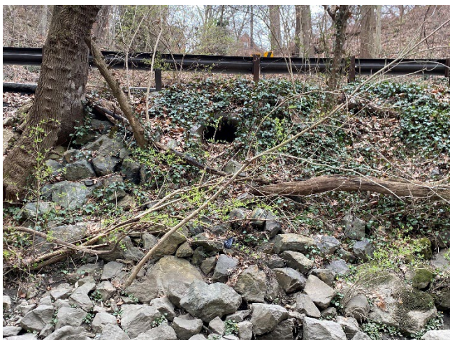
Photo 26 – Structure #986: Outfall overgrown with vegetation
