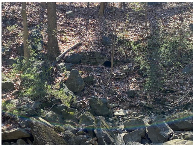
Photo 28 – Structure #1004: Outfall filled 35 percent with sediment and debris
