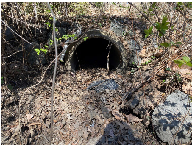
Photo 18 – Structure #273 – Outfall partially filled with sediment
