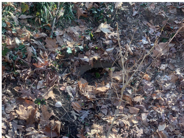
Photo 29 – Structure # 991: Outfall filled 95 percent with sediment and debris (don't have pic from this year)
