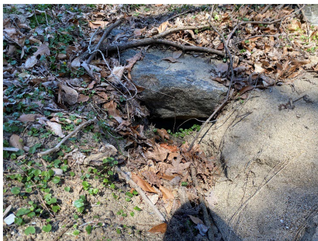
Photo 31 – Structure #1005: Outfall 95% full of sediment
