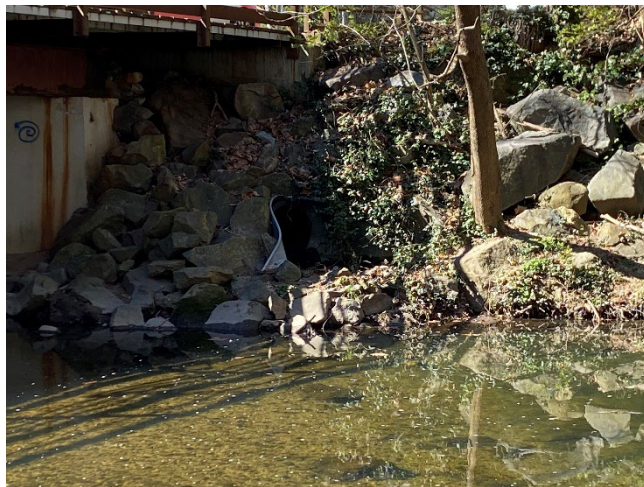
Photo 27 – Structure #983: Base is eroded
