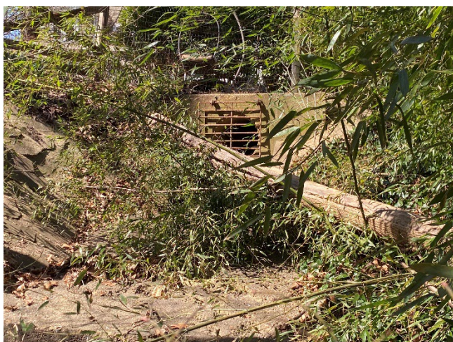
Photo 30 – Structure #1028: End of concrete channel undermined, 2-foot drop to channel along with eroded banks
