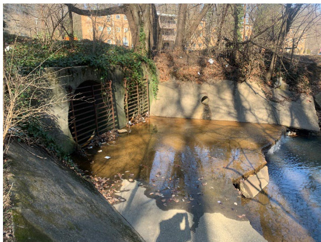
Photo 19 – Structure #289 & #290: Concrete apron cracked and undermined with deep scour pool; wingwall is cracked
