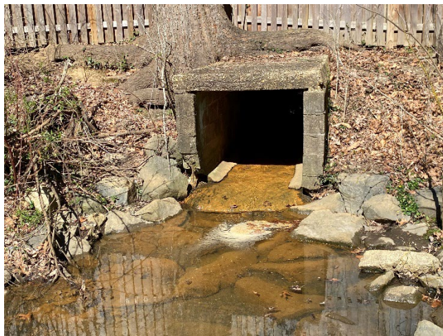
Photo 17 – Structure #212 – Corner of outfall broken
