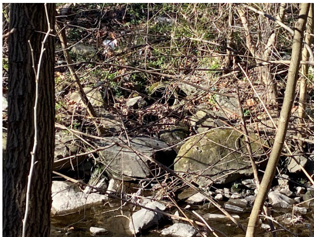
Photo 20 – Structure #854: Outfall is filled with sediment and leaf matter
