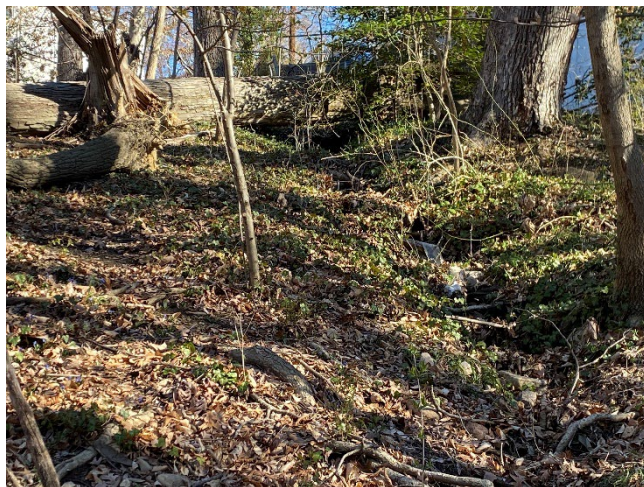
Photo 25 – Structure # 973: Outfall overgrown with vegetation and pipe broken
