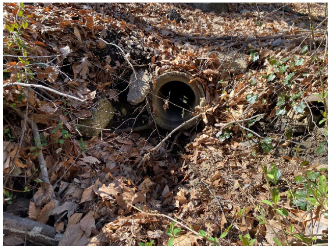
Photo 23 – Structure #960: Outfall has erosion under the pipe, has headcut and eroded banks leading to stream
