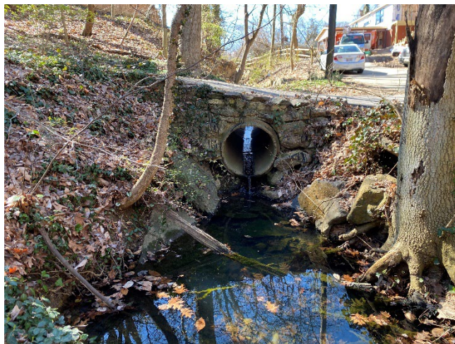
Photo 21 – Structure #881 is cracked on bottom causing erosion under pipe
