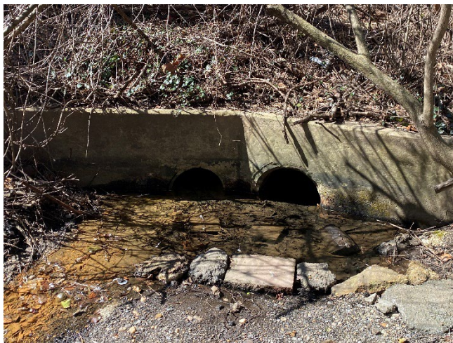
Photo 16 – Structure #71: Outfall 50% clogged with sediment
