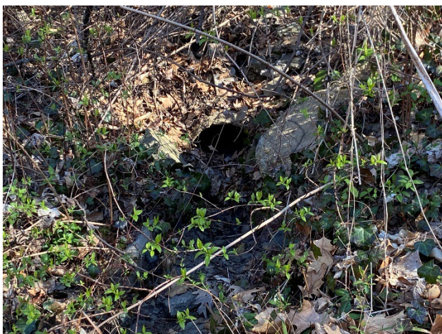
Photo 24 - #979: Obstructed by concrete and debris
