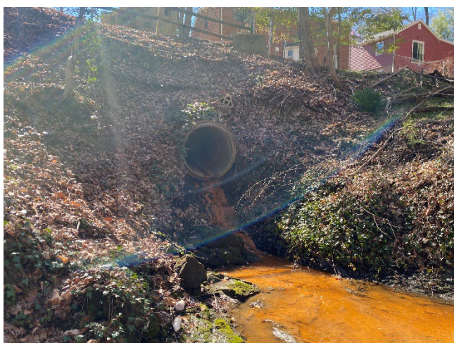
Photo 32 – Structure #1107: Crack in the pipe causing water to flow under the outfall causing erosion beneath the pipe
