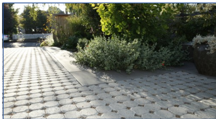
Permeable paving systems allow infiltration of water. Image credit: Landscape East and West
