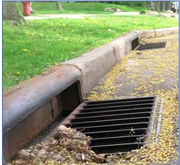
The public storm drain system is designed to carry stormwater away from developed areas and prevent flooding. Image Credit: MinnPost – www.minnpost.com
