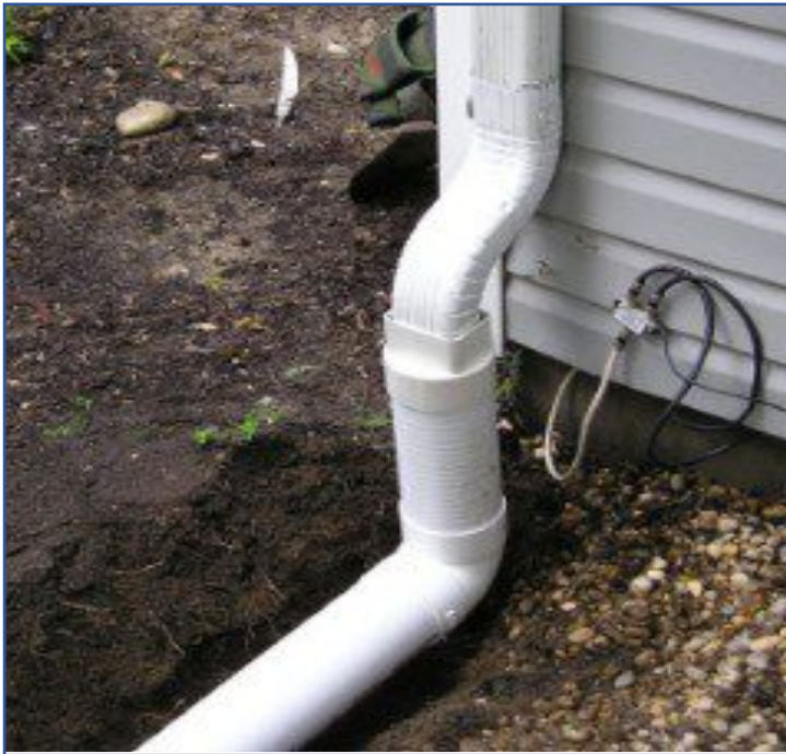
Leader pipes can be used to extend downspouts beyond building foundations. Image Credit: LID Center
