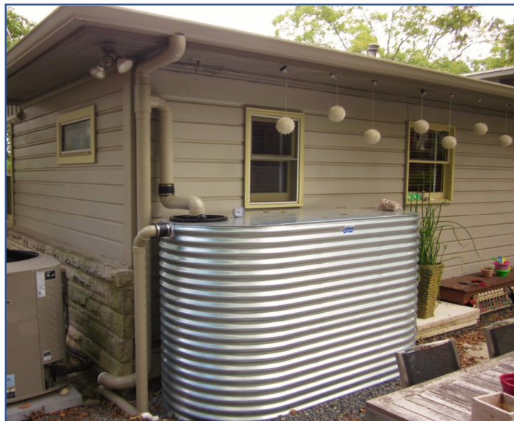
Cisterns can be used to harvest and utilize rainwater. Image credit: Innovative Water Solutions – watercache.com
