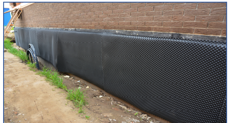
Exterior waterproofing membranes protect a home's foundation from groundwater intrusion.
