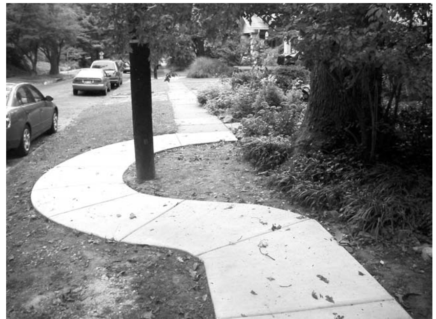
Throwing a curve: on 7300 block of Willow Ave., Public Works tailors the sidewalk to protect tree roots.
