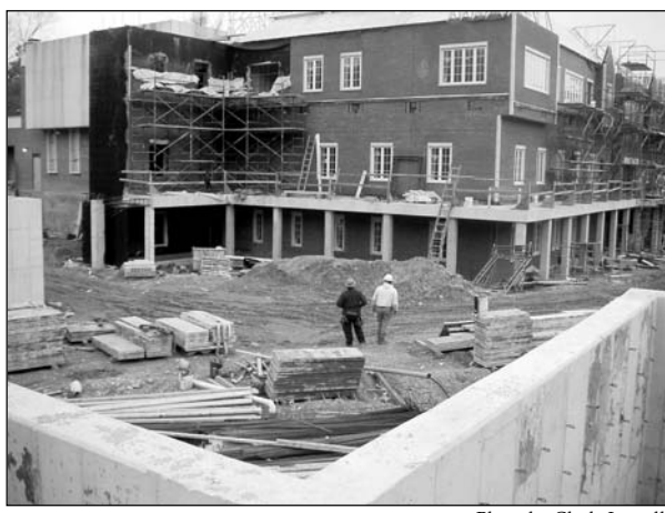
Photo by Clyde Lassell Community Center construction, January 2005
