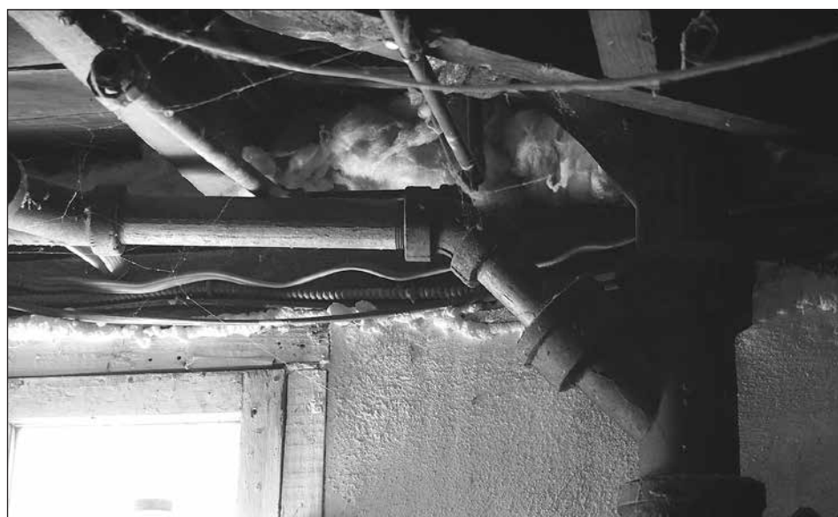
Basement: The band joist line in the basement was sealed with spray foam, along with other draft sources throughout the home to prevent air leakage.
