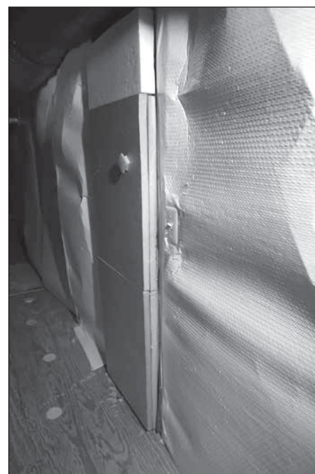
The door to the 2nd floor crawl space (kneewall) as well as the walls were insulated and sealed, and small holes drilled into the floor so that dense pack insulation could be sprayed in.
